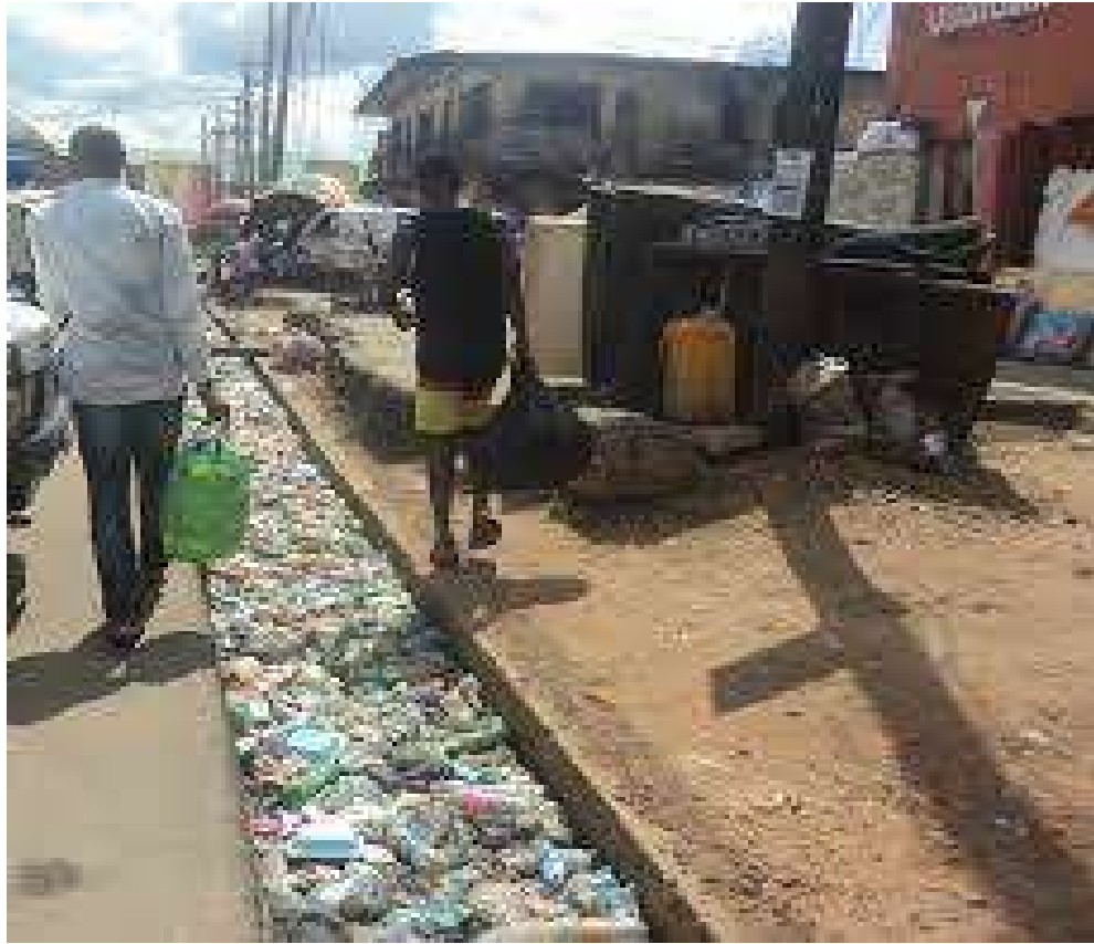
Figure 1: Photograph of Polythene waste blocking drainage Source: [8]
